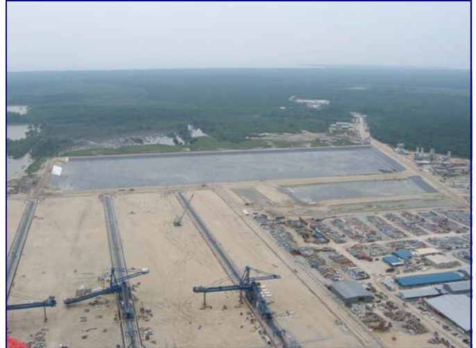
The first square meter of the 2.00mm GSE geomembrane was laid on Sept. 30, 2005. By Nov. 30, 2005, 201,000 sq.m. were laid, seamed and tested. Of these 60 days, it rained at least 30. Work has slowed down since the end of November 2005 due to interruption around concrete structure areas like cascading drains, pipe penetration and pump sumps.
